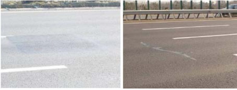
Fig. 1. Pavement cracking
